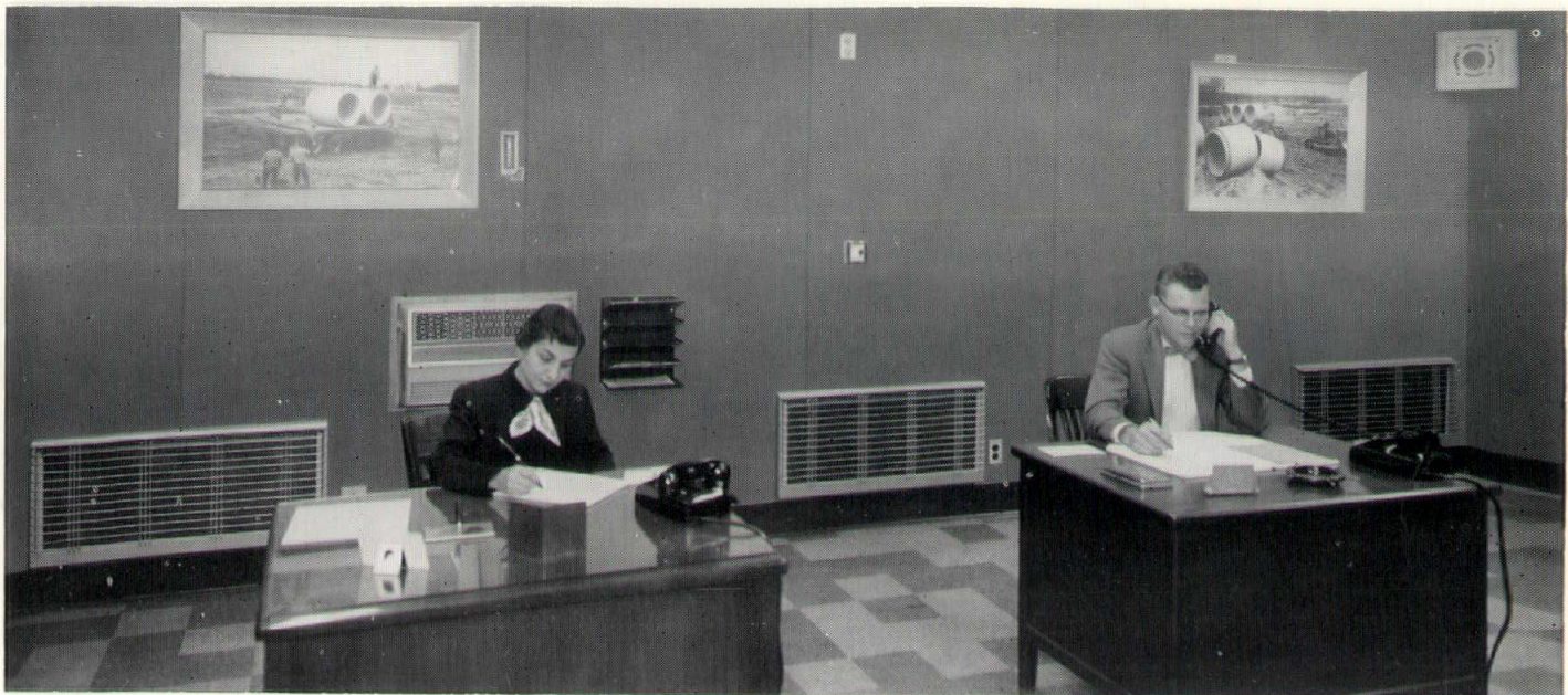
Office of Mr. Squires and secretary Isabelle Johnston at the Superior Products plant, showing space-saving installation of electric heaters in the rear wall.
