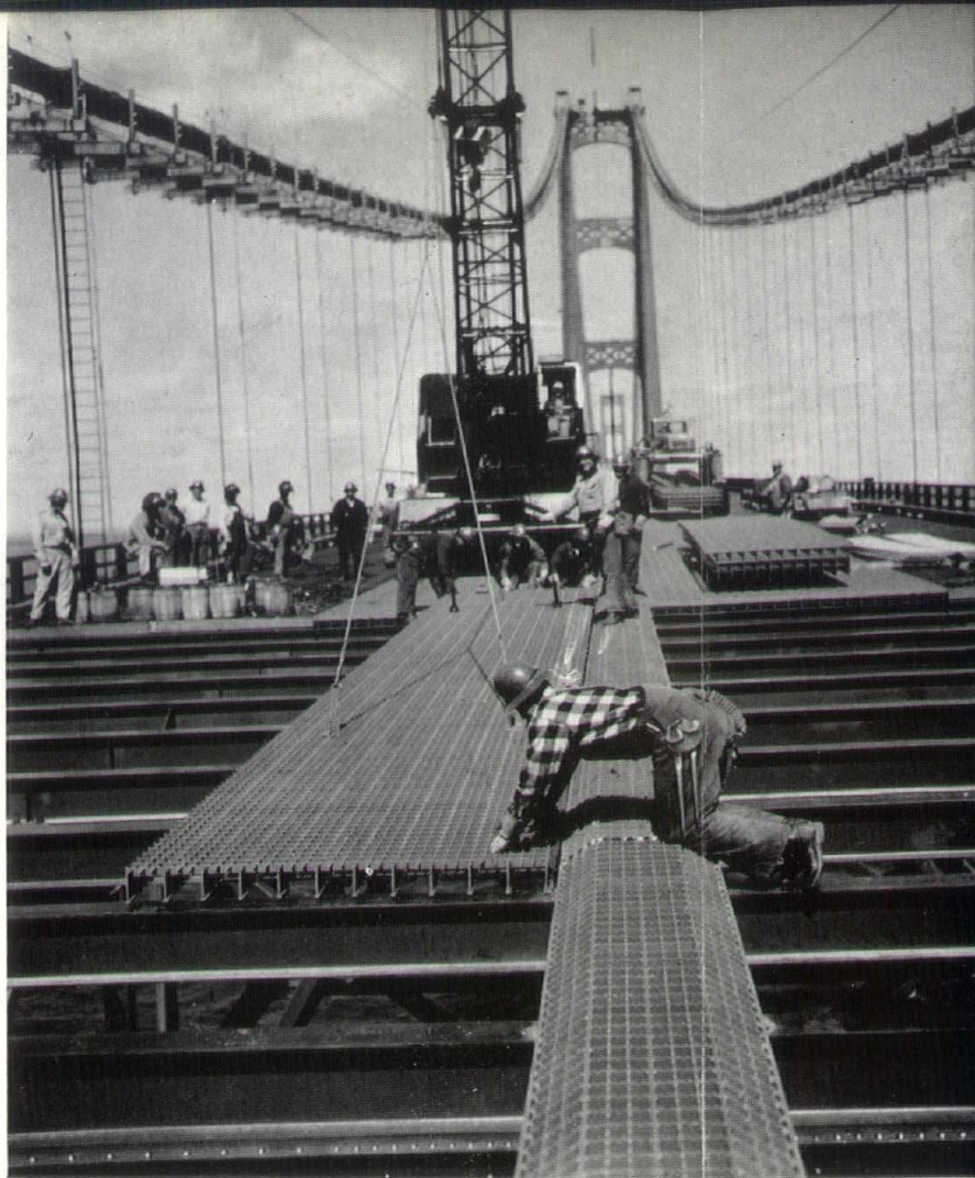
LAYING I-BEAM-LOK STEEL FLOORING
