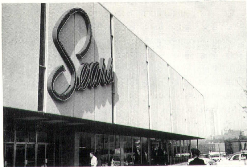
Modern architectural beauty is achieved with Marietta precast wall panel construction in a Nashville, Tenn. shopping outlet
