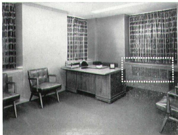
Flush wall unit in doctor's office.
