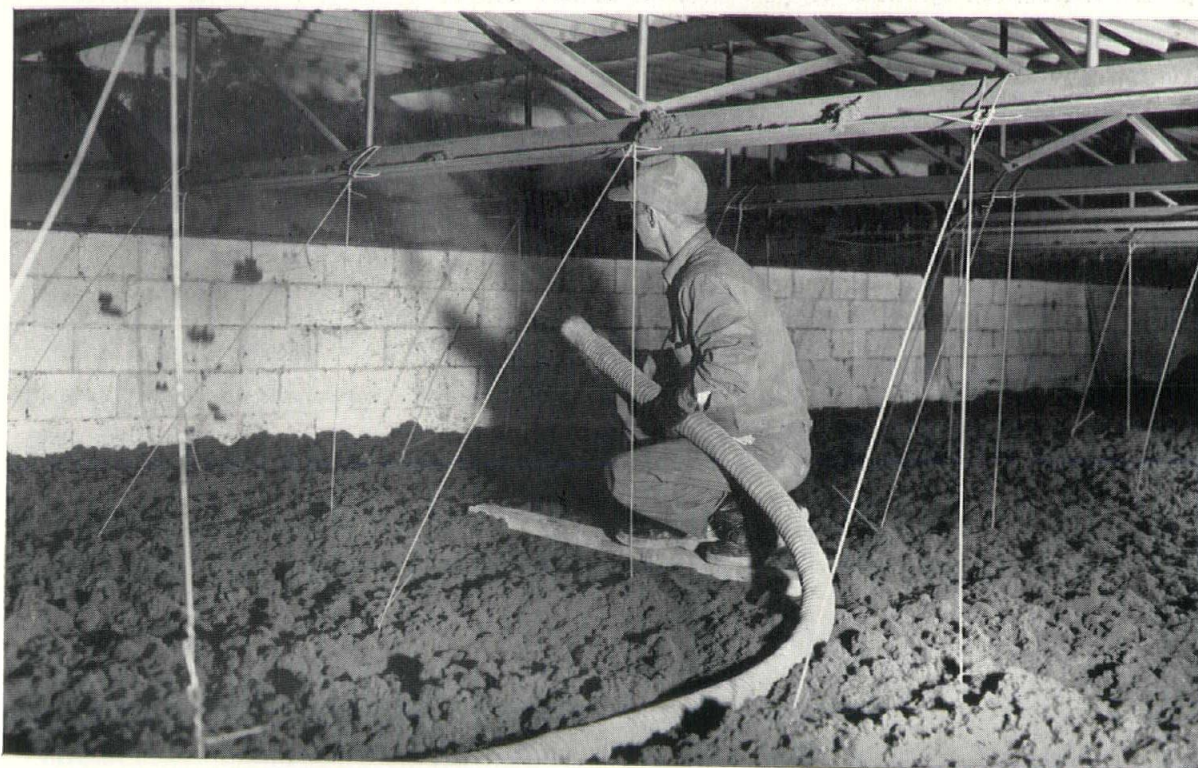
Coefficients of Transmission (U) factor of this ceiling, .069 with 4 inches "Silvawool"
