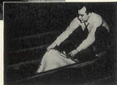
Photo of cotton insulation after bad fire.
