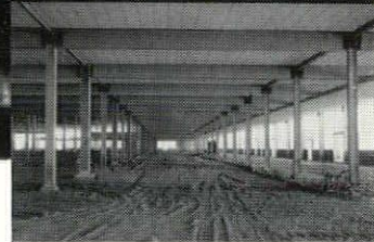
Flexicore mezzanine at new Rex Manufacturing Co. plant, Connersville, Ind., is 760' long, 115,000 sq. ft. of slabs used.
