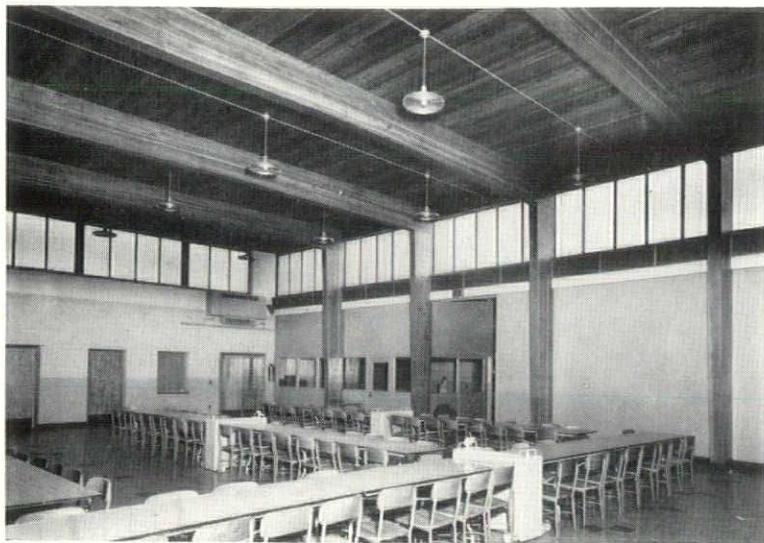
Cafeteria of Centerline High School, Centerline, Michigan, is 66'-8" x 62'-4". Glulam timber girders resting upon glulam columns are spaced at 12 feet. Architect: Brender & Van Reyendam, Detroit; Atkin-Fordon Co., Detroit, is general contractor.
