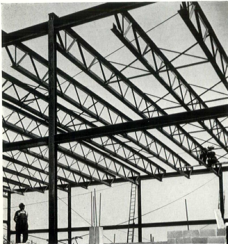
The roof construction of this Grand Haven Senior High School building uses 81-foot T-Chord Long Span Joists. Architect: Warren S. Holmes
