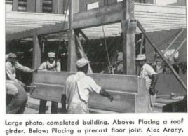
Large photo, completed building. Above: Placing a root girder. Below: Placing a precast floor joist. Alec Arany, engineer; John K. Minasian, consulting structural engineer; J. A. McNeil Company, Inc., contractor, all of Los Angeles.
