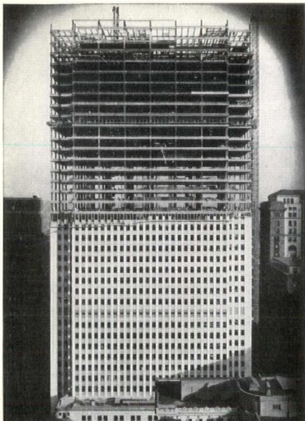
At Pittsburgh's newest skyscraper, the 525 Wm. Penn. Place Building, Robertson Q-Floor construction has simplified and speeded the work of every sub-contractor. Each floor is a clean, uncluttered, available working area.
