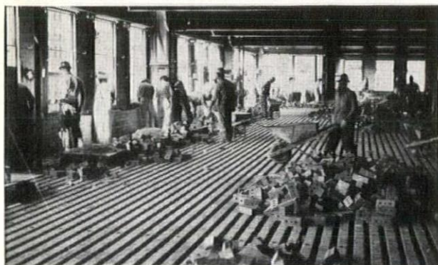
No forms or shoring to hinder them, each trade can work safely with materials and equipment immediately loaded on the Q-Floor. No need to use streets or sidewalks for storage.
