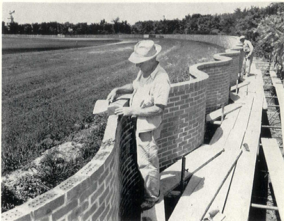
This mile-long serpentine brick wall is being built along the Village Road side of the Ford Motor Company's test track in Dearborn. One brick thick, it is built on a concrete footer two feet wide and three and one-half feet thick.
