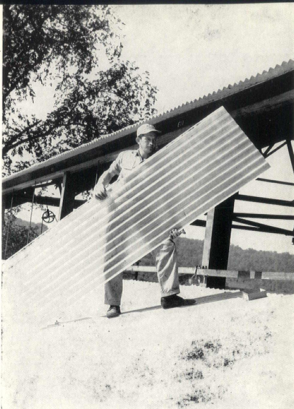
Resolite Corp., Zelienople, Pa., is producing translucent structural panels, reinforced with fiberglas mat. Sheets come in six colors, and, in addition to flats, are molded in all standard roofing sheet corrugation sizes.
