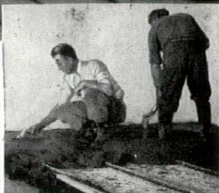
Covering Coils with Ordinary Concrete.
