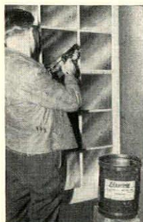
Caulking Gun with Special Nozzle used to apply Bedding Cement
