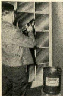
Caulking Gun with Special Nozzle used to apply Bedding Cement
