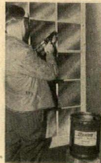
Caulking Gun with Special Nozzle used to apply Bedding Cement
