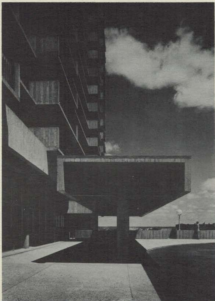
VISTA DEL RIO, Kansas City, Missouri. ARCHITECTS: John Lawrence Daw & Associates, Architects & Planners, Kansas City. GENERAL CONTRACTOR: J. E. Dunn Construction Co., Kansas City. Dover Elevators Installed by Dover Elevator Co., Kansas City.
