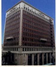
110 PINE AVENUE BUILDING, LONG BEACH Hundreds of bricks were replaced, and repointing was done. Terra cotta pieces were removed and reassembled. Stainless steel rods set in epoxy were used for added strength.
