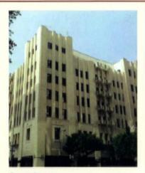
CARRIER CENTER (formerly Robinson's Department Store), Los Angeles. More than 2,000 ceramic tiles and terra cotta blocks were removed, replicated, and replaced. 500 double hung windows were restored.
