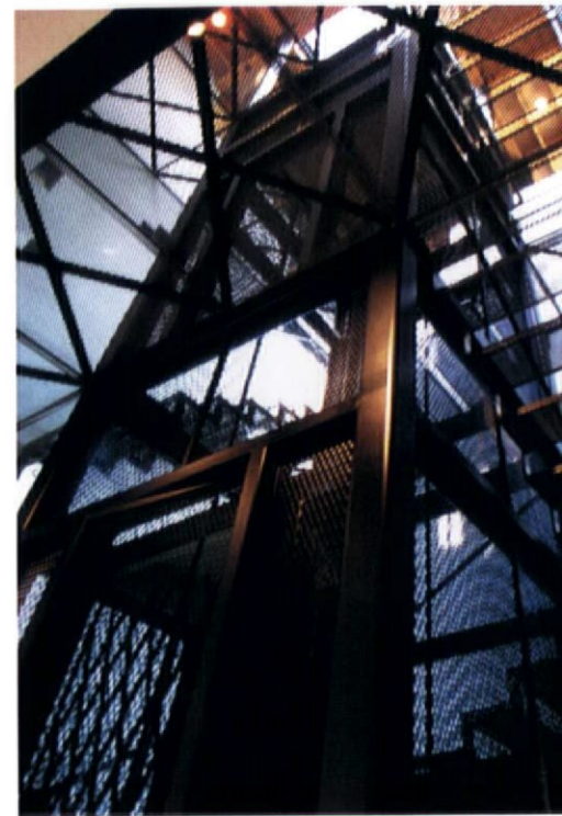
The 40' perforated steel, woven wire fabric and mesh stair and elevator core creates an open shaft which is used as a solar chimney to exhaust and recover heat which collects at the high ceilings of the living room and master bedroom.
