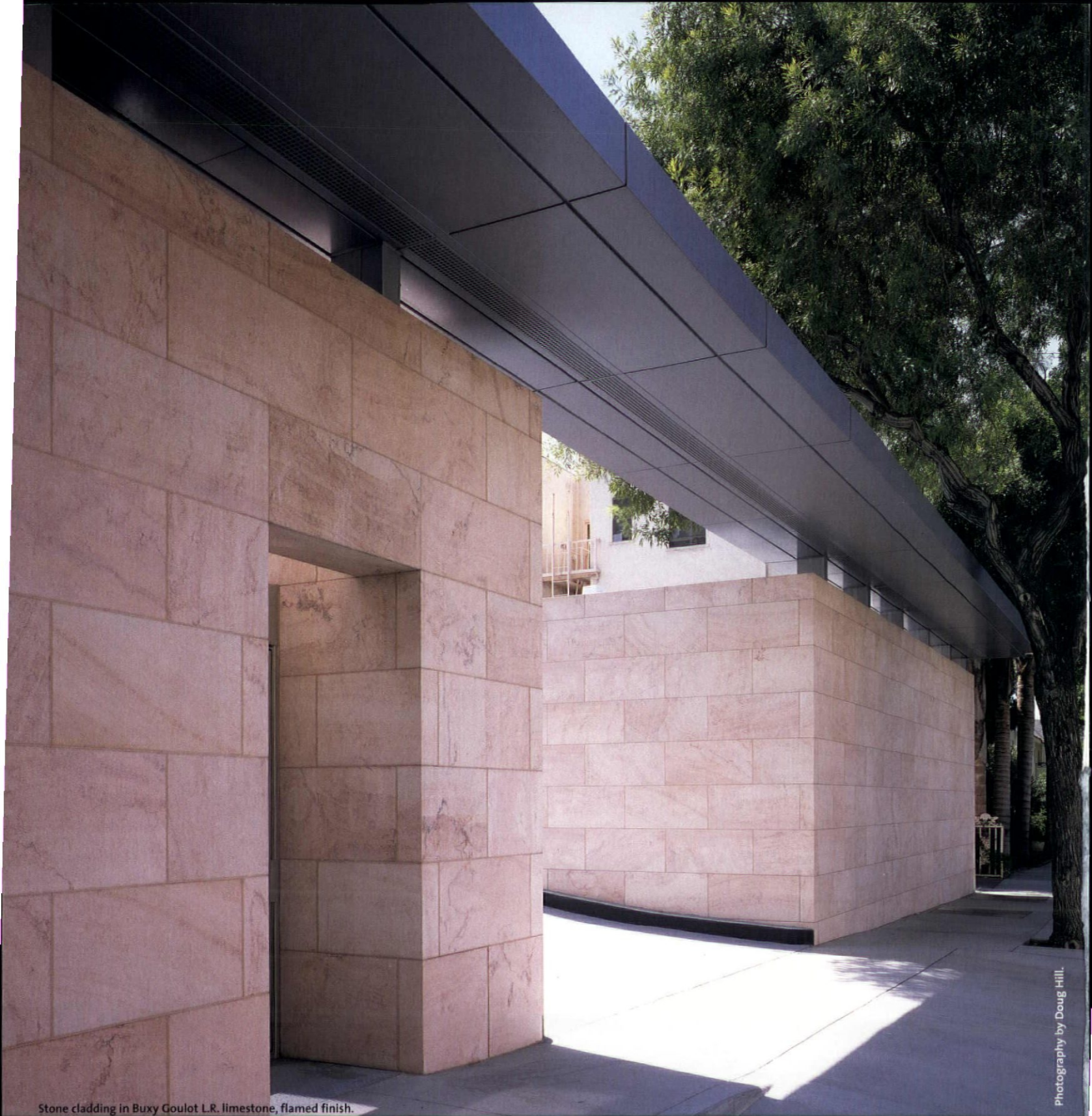
Stone cladding in Buxy Goulot L.R. limestone, flamed finish.
