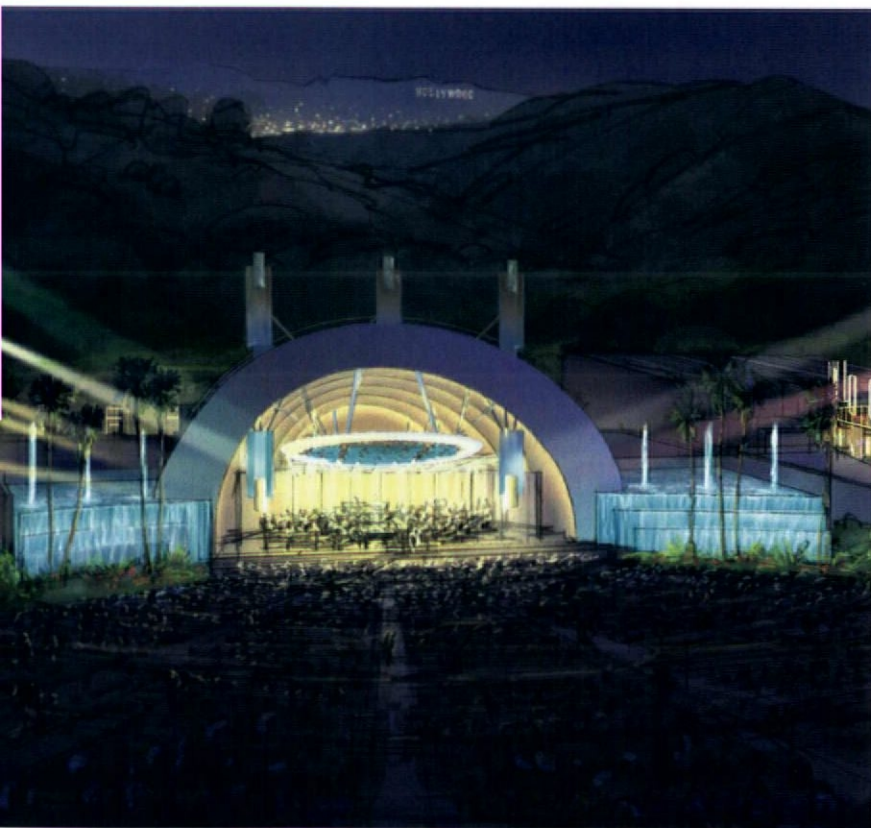
HOLLYWOOD BOWL—Above: The new shell by Hodgetts + Fung. No stranger to replacement, the present shell is the fourth one built. Hodgetts + Fung's new, larger shell will house a technological marvel—an "acoustical cloud" that will hang thirty feet above the performers and will bounce sound back uniformly. The disc will even adjust to atmospheric changes at the outdoor venue. Left: The "acoustical cloud" or disc.
