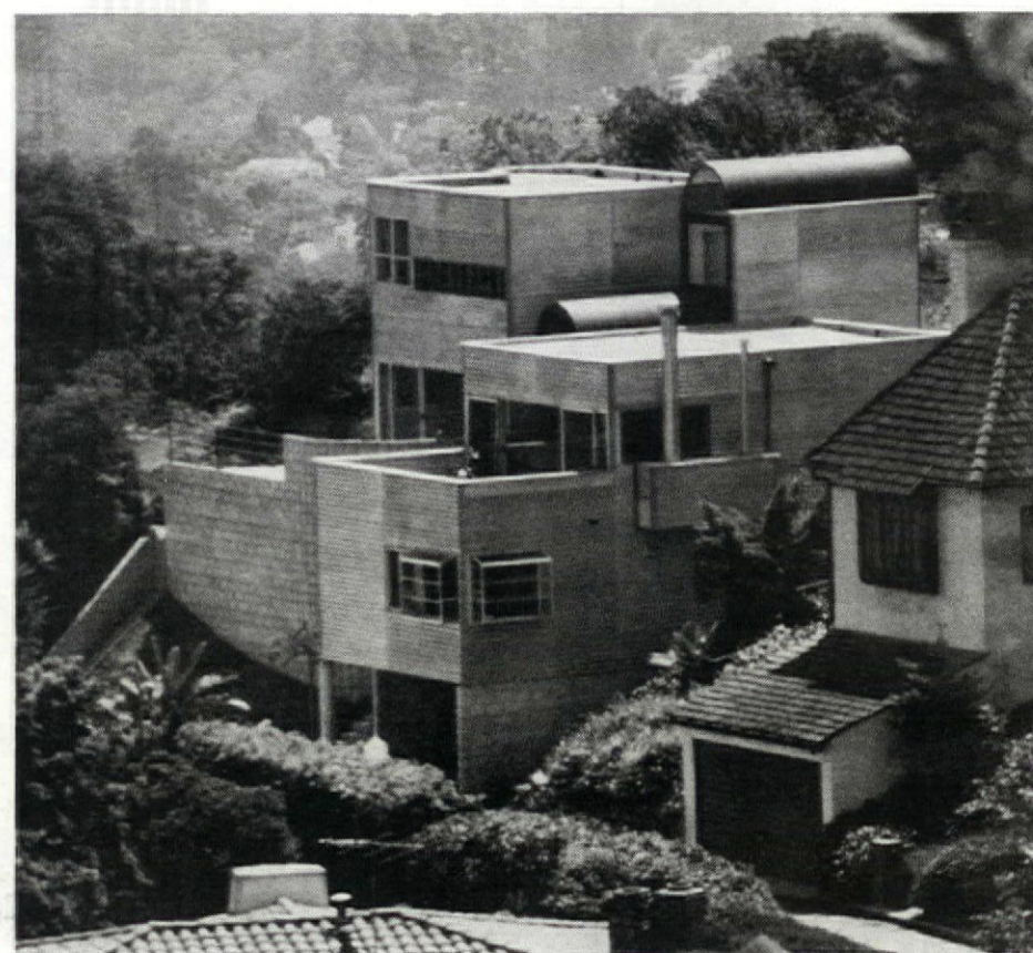
House by Mark W. Hall uses prefabricated silo walls for its structural system.
