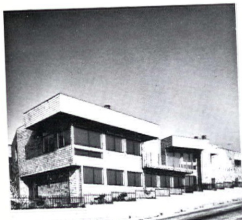
Elster beach front speculative house, above, 1979, Playa del Rey. This house was built on an "impossible" lot. The foundation bridges across a 30 ft. easement and avoids any surcharge on the deeply buried culvert. A cantilevering retaining wall on cantilevering grade beams was the solution for the narrow wing which could not bridge the easement because of setbacks. The Coastal Commission limited the height to 3 ft. above the upper street to preserve a public view of the ocean.
