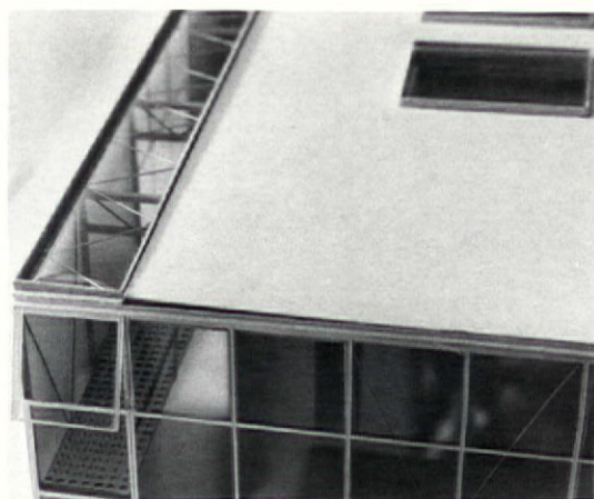
Detail of the de Bretteville house North wall Studio shows skylight and horizontal Trussjoist.
