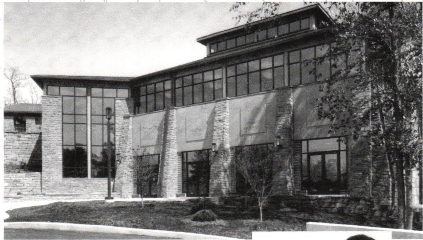
Merit Award - Ratio Architects, Inc. for Brown County Public Library in Nashville, Indiana.
