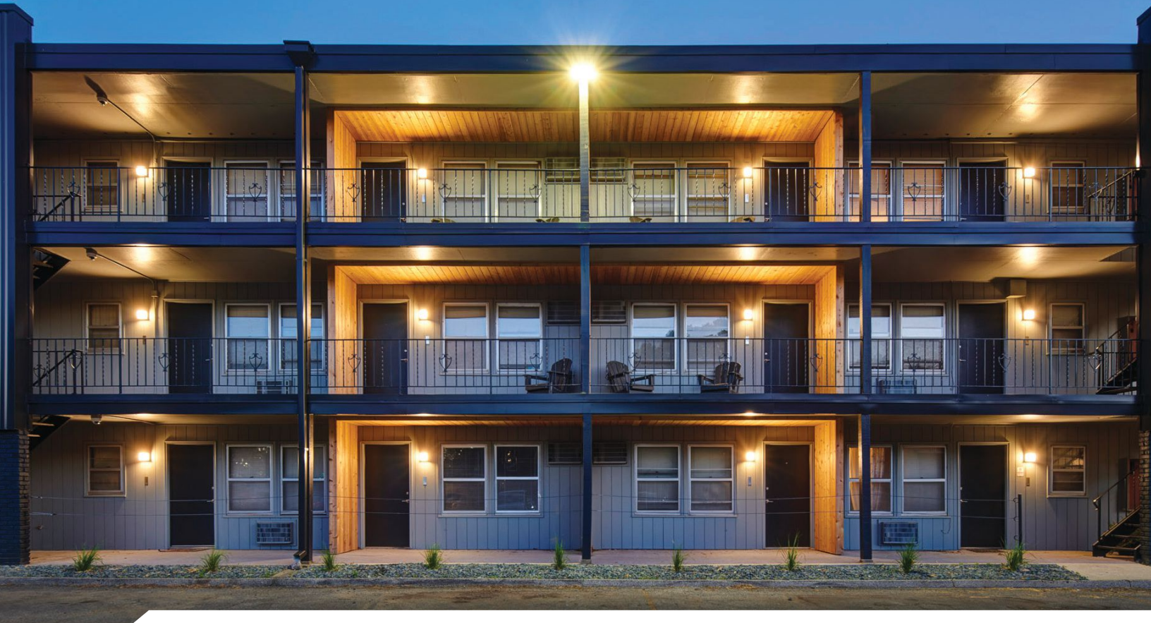
Above: Existing upper floor railings were updated in black to recede from new exterior wood elements.
