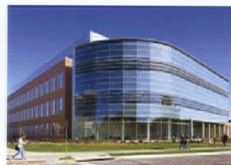
Iowa State University Hach Hall Chemistry Building - Ames
