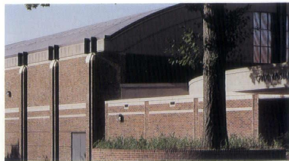
A sweeping stucco fascia encircles the existing auditorium and marks a secondary entry linking the gym to the original school.
