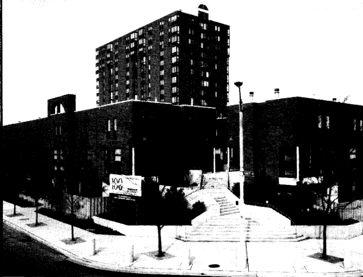
100 Forest Place Architect: Phillip Kupritz & Associates Mason Contractor: J & E Duff
