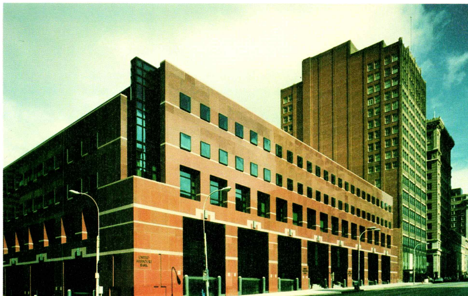
▼ Red granite and black stainless steel columns surround the building and line either side of the deep narrow alley which leads to the street.
