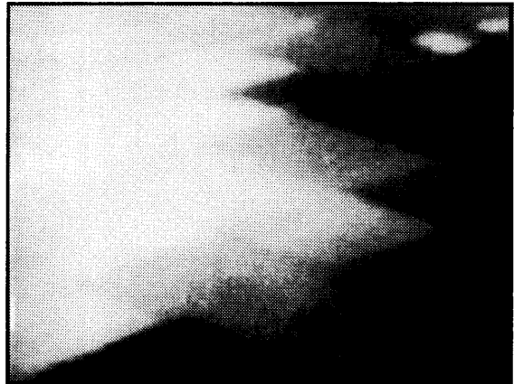
Wet insulation as seen in infrared.
