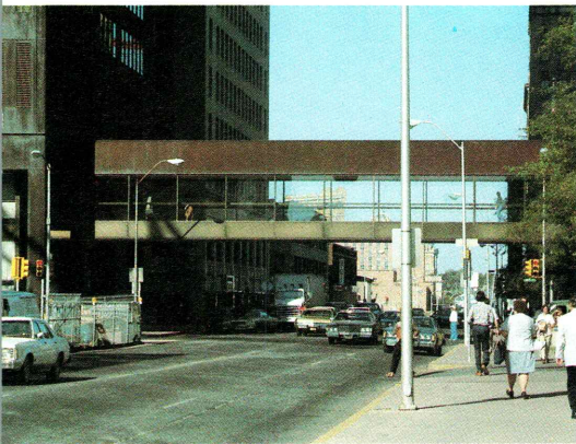
The Skywalk spanning Grand Avenue to the Ruan Center, completed in 1974, was a private bridge connecting to a public parking garage. The City of Des Moines purchased this Skywalk to incorporate it into the public system in 1981.
