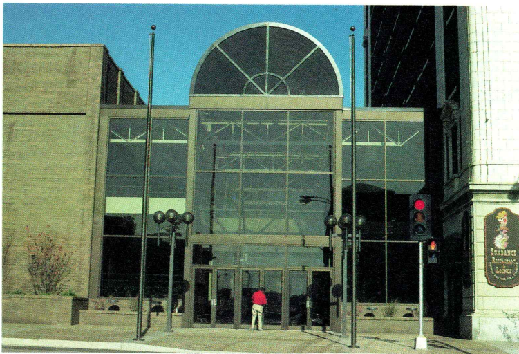
Above and right: The glass-enclosed lobby, the building's centerpiece, ties the exhibition area to the Blackhawk Hotel and overlooks the Mississippi River.
