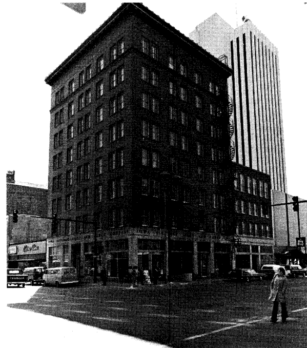
Security Savings Bank Building (Iowa Electric Light and Power Company), Cedar Rapids. Conversion of this building for use as a department store involved minimal exterior restoration as the exterior had been well-maintained over the years. Photo: Iowa State Historical Department, Division of Historic Preservation.
