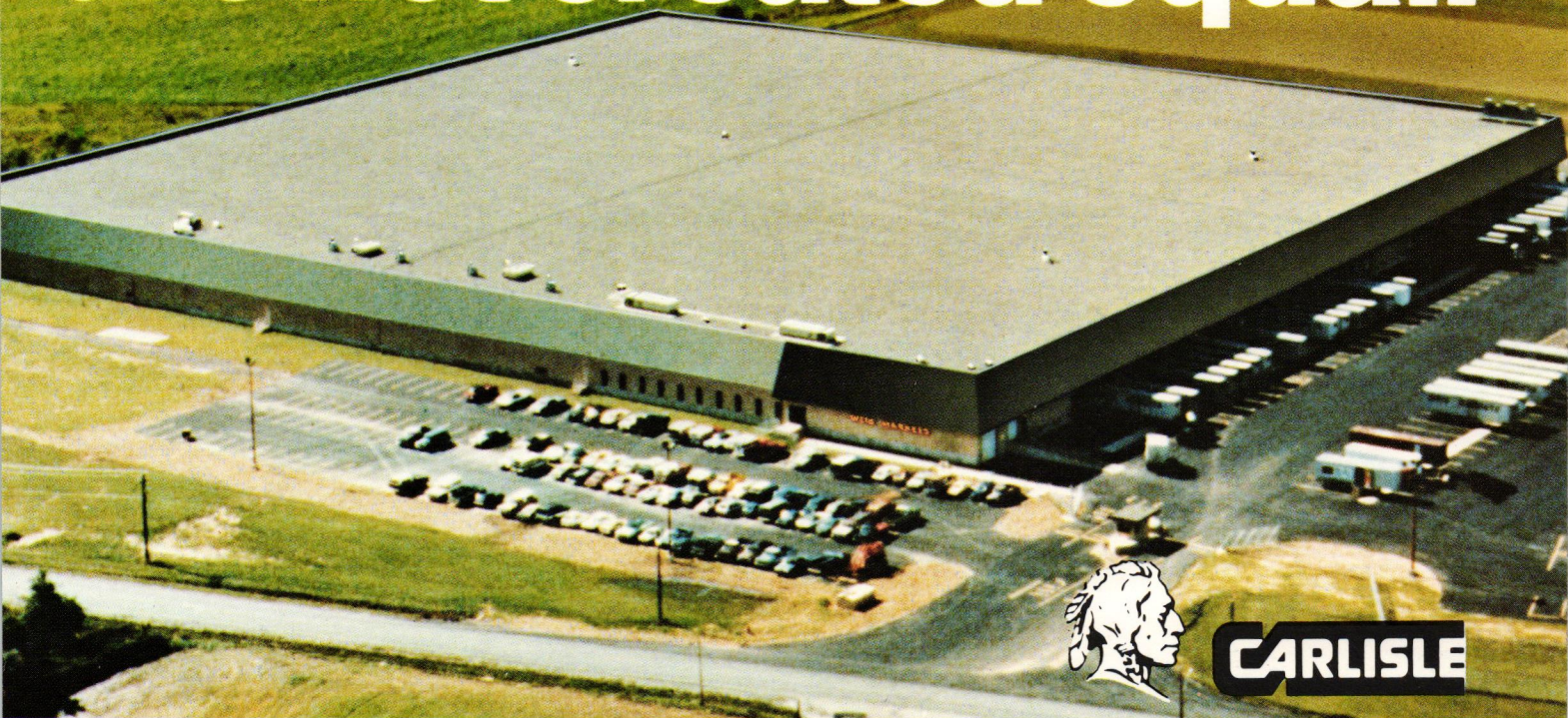
Aerial view of the Carlisle roof on the new Milton, Pennsylvania Distribution Center
