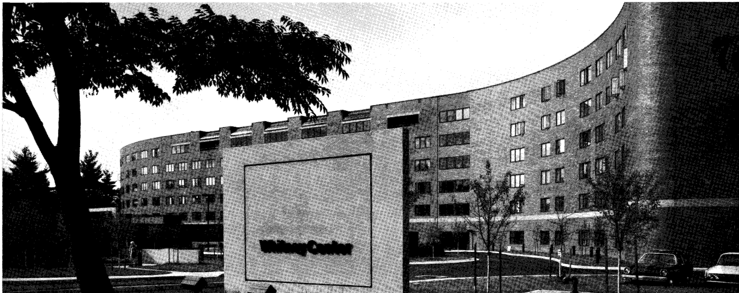
23. 1979 Award of Excellence Whitney Center, Elderly Care Facility Hamden, Connecticut Engelbrecht/Rice/Griffin, Architects Photo: Julius Schulman
