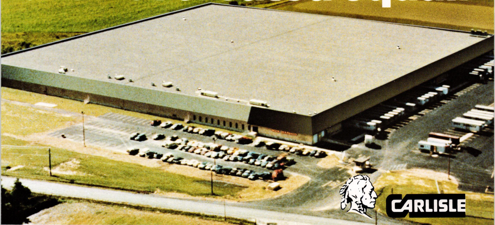
Aerial view of the Carlisle roof on the new Milton, Pennsylvania Distribution Center
