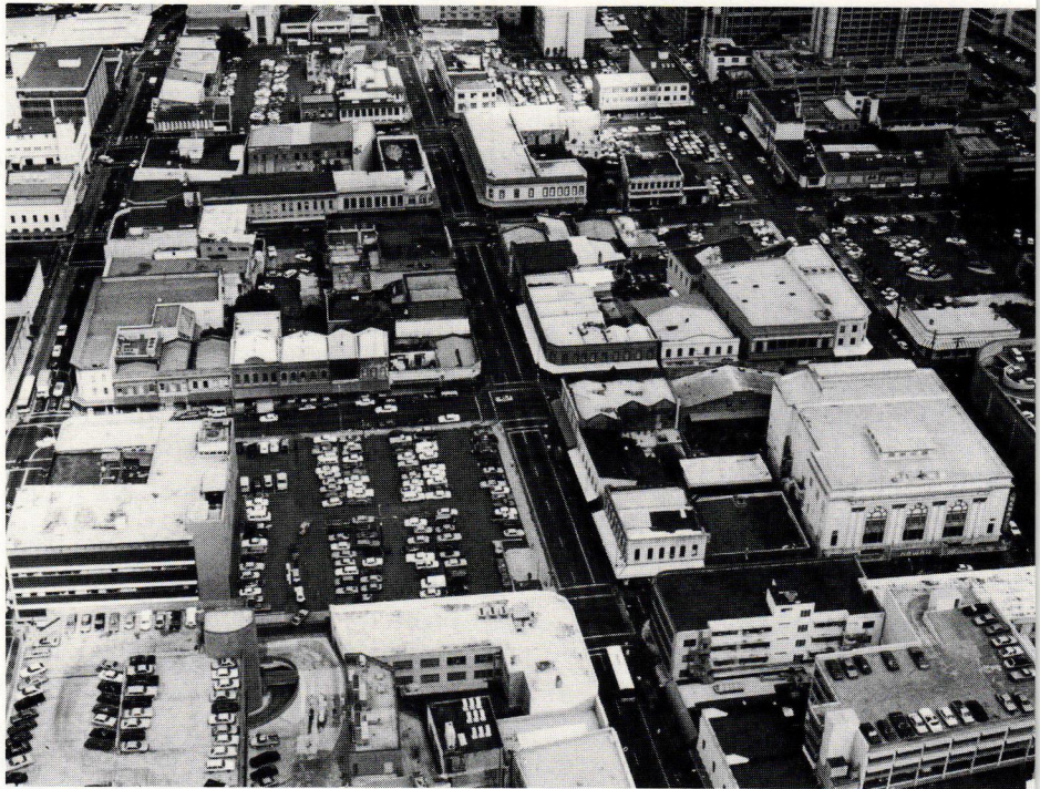
An overall view of the Chinatown District where the $25 million Chinatown Gateway Plaza project is planned. Photography by Tom Hisamura and Ben Lee.
