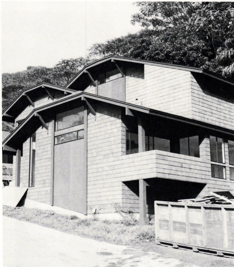
Wood double-wall framed gypsum interior with external siding. A design and form, using an accepted building technique. Photos by Jeff Nishi
