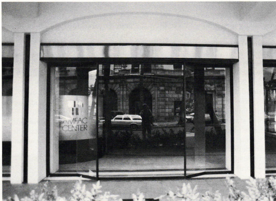
A new look at the AmFac Center shop fronts was achieved with stainless steel and satin bronzes combined with mitered glass.
