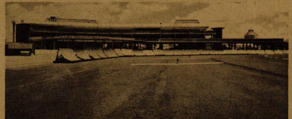
Atlas Electric installed 22 Montgomery escalators and 15 elevators at expanding Honolulu International Airport.
