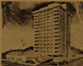
Two high-speed Montgomery elevators are installed in the Kealani, a 15 story highrise on the Ala Wai.
