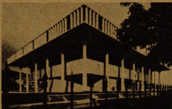
The Hawaii State Capitol Building utilizes 7 Montgomery elevators.
