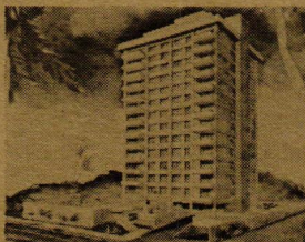
Two high-speed Montgomery elevators are installed in the Kealani, a 15 story highrise on the Ala Wai.
