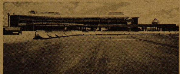
Atlas Electric installed 22 Montgomery escalators and 15 elevators at expanding Honolulu International Airport.
