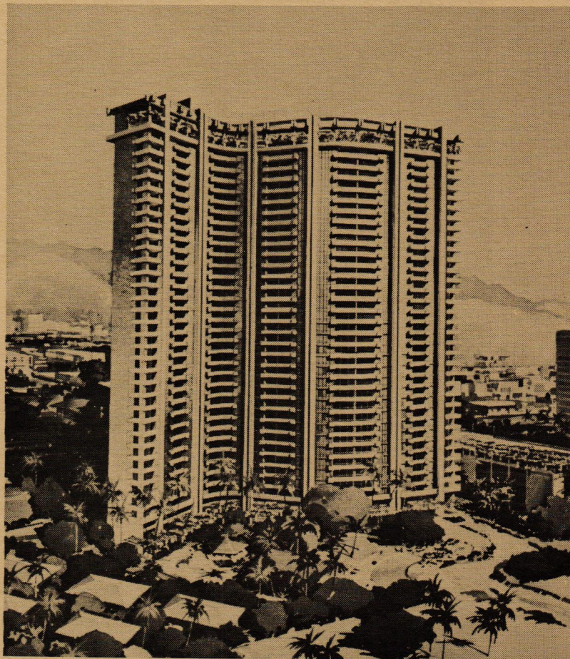
Owner-Developer: Reed & Martin Investment Corp. Architects: Lemmon, Freeth, Haines & Jones John Carl Warnecke & Associates Walter K. Tagawa & Assocs., Inc., A.I.A.
