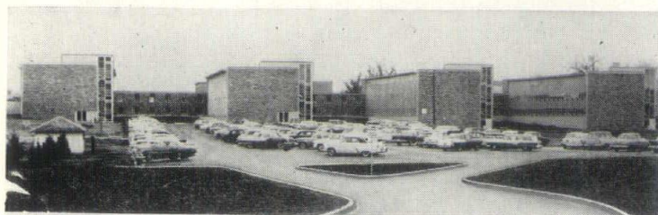
12,200 square feet of Porcelo Panels were used in the construction of the New Engineering Building at Colorado A. & M. College.
