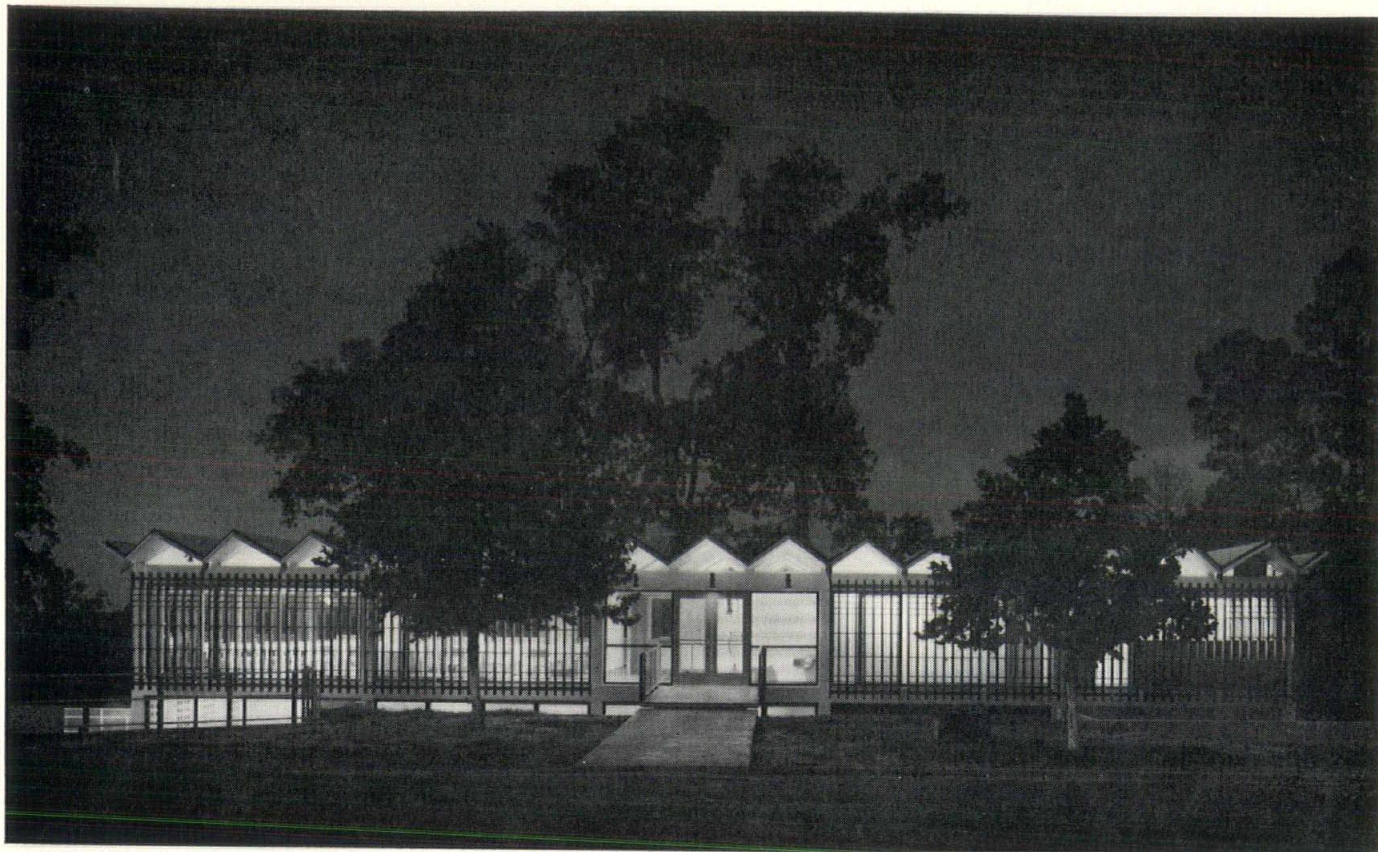
Front Elevation Restaurant Building, Hot Wells, La.
