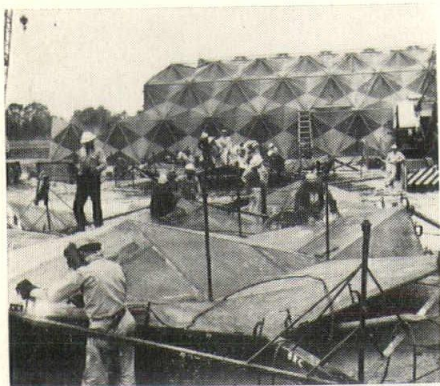
Welders begin fabrication of a steel section on the ground at job-site (above). Cleaning and coating prior to placement is performed by section being placed on steel rack (below).
