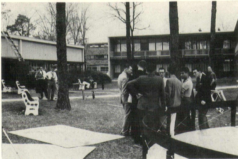
Students on the LSU Department of Architecture tour of Houston construction, at the site of the Buckminster Fuller geodesic dome being built on the University of Houston campus. Sheets on ground are for plexiglass skin of dome.
