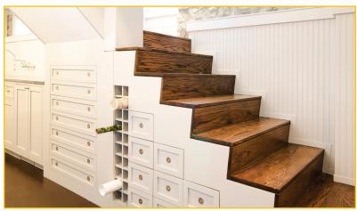
Detail view of the staircase with integral storage.
