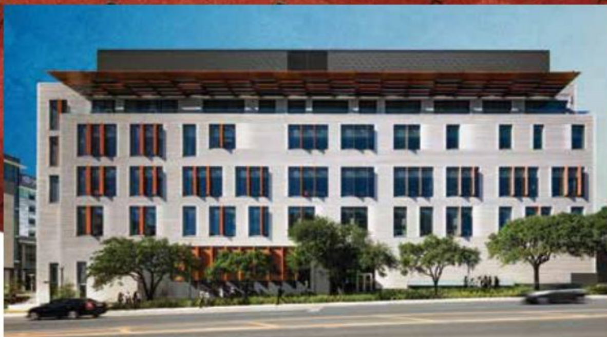
Dell Medical School Health Learning Building, designed by Page, located between the Texas Capitol and I-35 / Photo: Albert Vecerka/ ESTO Photographics
