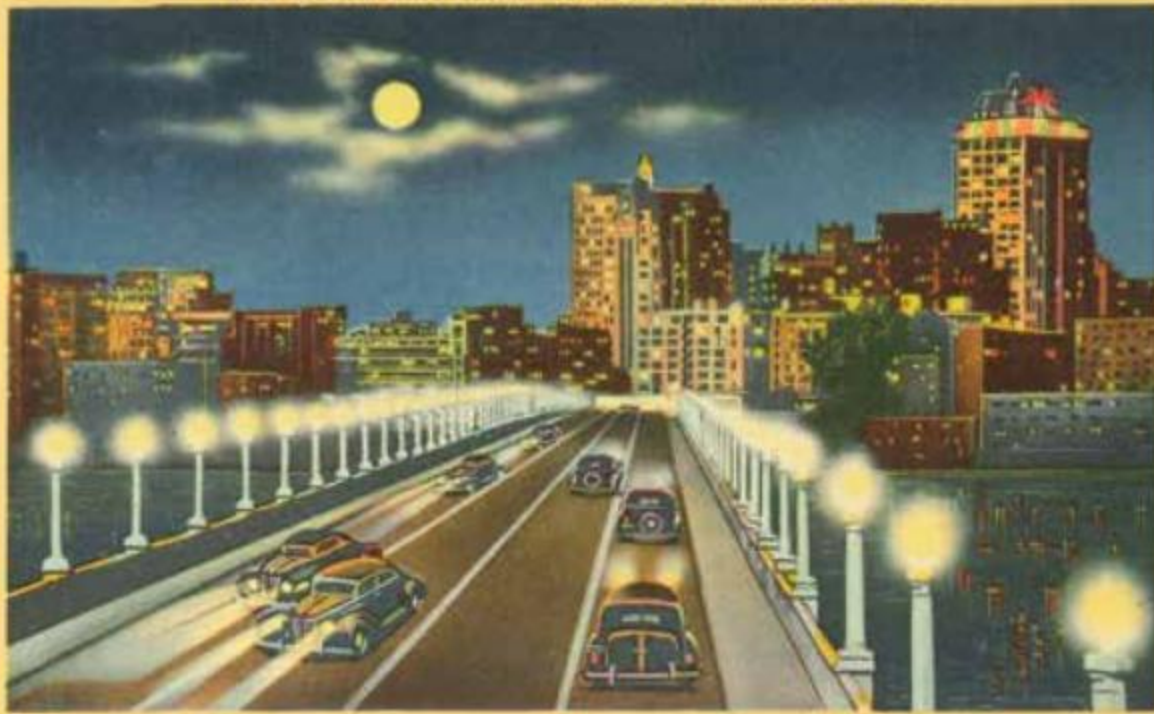
D-41—Houston Street Viaduct and Skyline by Night, Dallas, Texas
