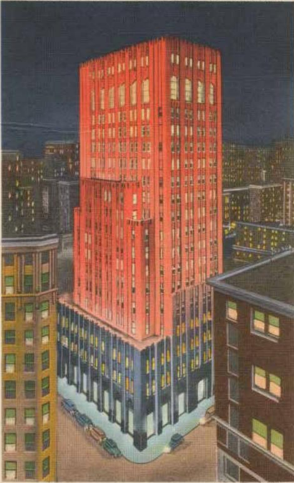
DALLAS POWER & LIGHT COMPANY. NIGHT SCENE, DALLAS, TEXAS
