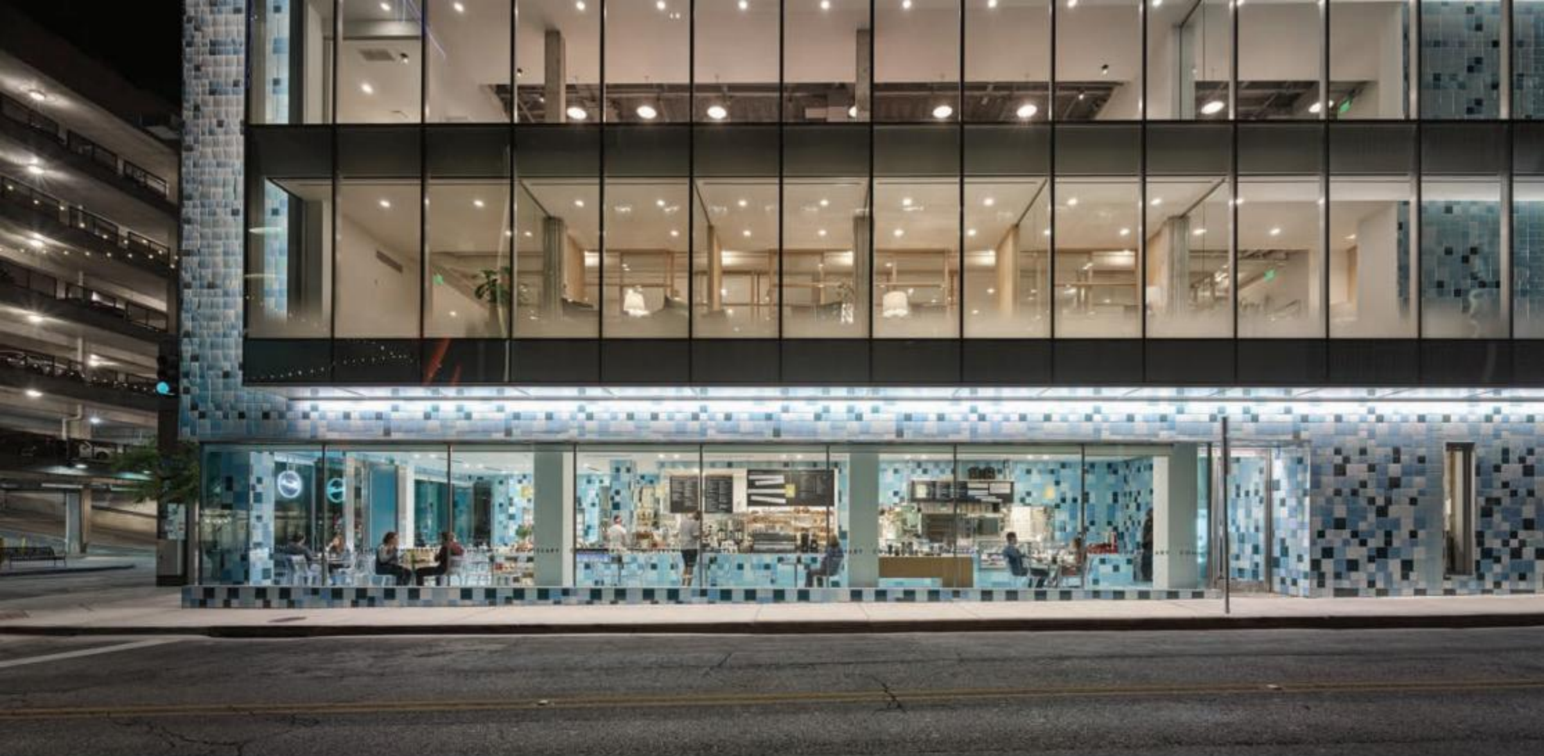
Medium Studio: The facade of 1217 Main Street in Dallas is a unique collaboration of 5G Studio Collaborative and artist Jorge Pardo. / Photo: Adam Mork
