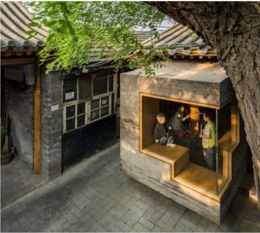
Above: A small plywood children's library sits among the residences created from a transformed temple in Beijing. This small-scale project has helped create a community bond among residents.
