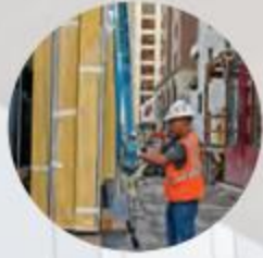
prefabricated exterior wall panels
