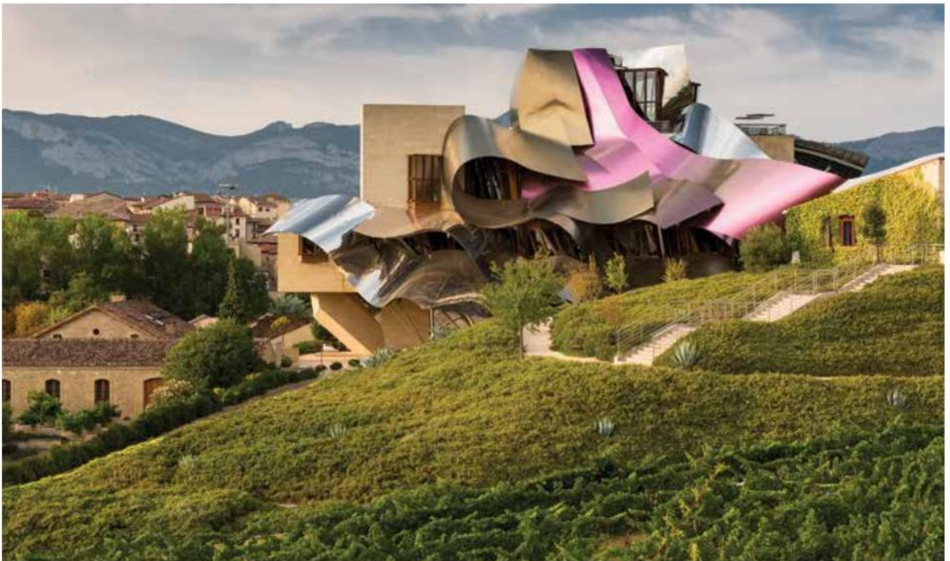
Hotel Marqués de Risca designed by Gehry Partners, LLP. An attempt at elegance is burdened by the weight of its own structure and the building underneath. / Photo by Adolfo Rancano/Marriott International
