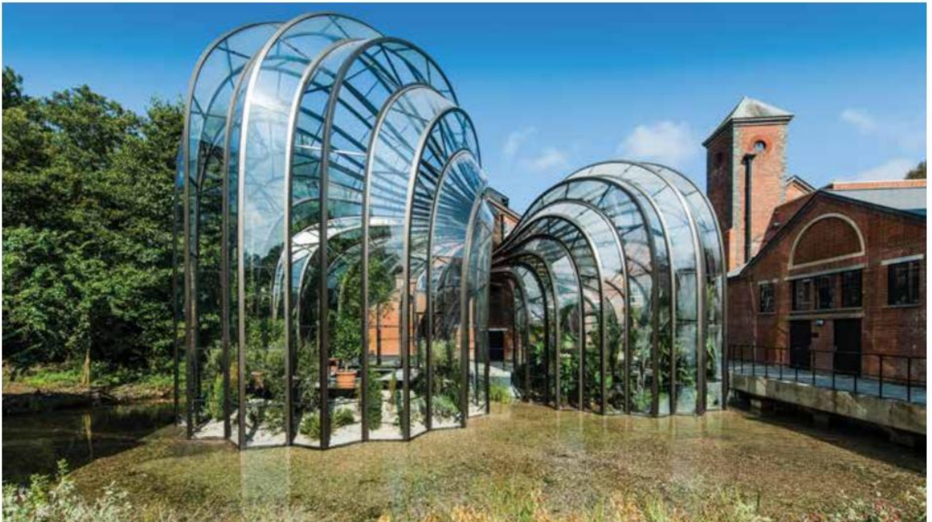
Bombay Sapphire Distillery designed by Heatherwick Studio. Glass ribbons and metal boning extrude from the apertures of an adjacent building. The structure is a nod to the 1854 Crystal Palace, and a comparison between the two show how far advancements in material fabrication, production, and design have advanced. / Photo by Iwan Baan
